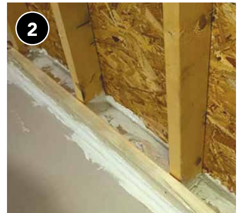
Ensure balloon-framed walls are blocked at top and bottom to prevent insulation from unintentionally blowing into the attic or basement.
