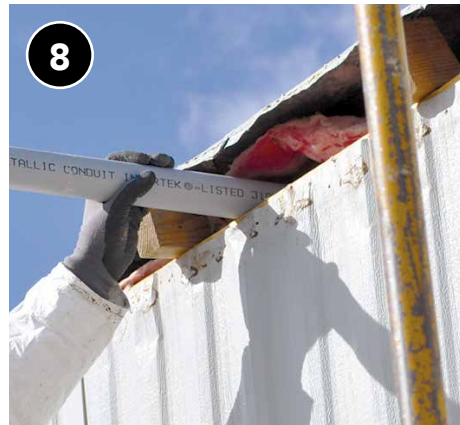
8 Insert blower hose as far as possible into cavity and retract slowly while filling space between trusses.
