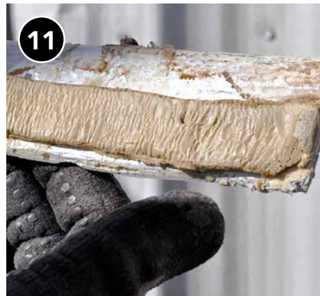
11 Replace butyl tape on J channel.
