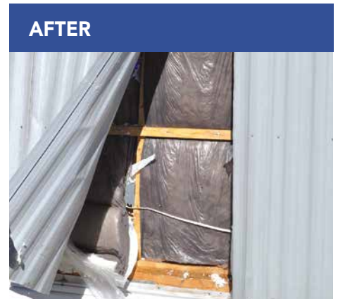
Properly installed insulation will have no gaps and minimal compression when complete.
