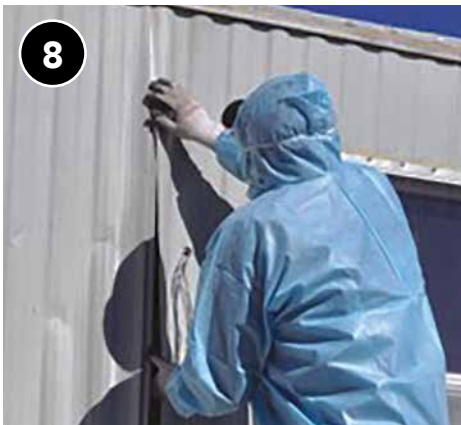
8 Carefully reinstall the siding.
