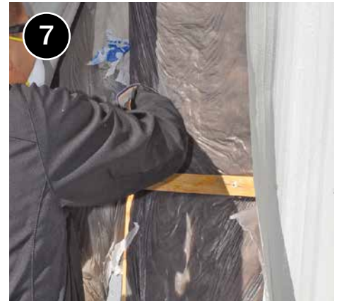
7 Gently tug batt into place, tuck remaining batt under lower belt rail, and fit down to bottom of cavity with minimal compression.
