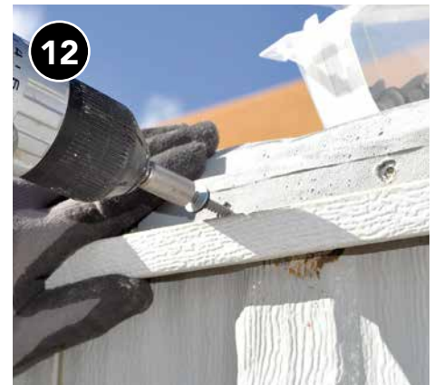
12 Reattach J channel, lapping over edge of roof. Repeat entire process for other side, if necessary.
